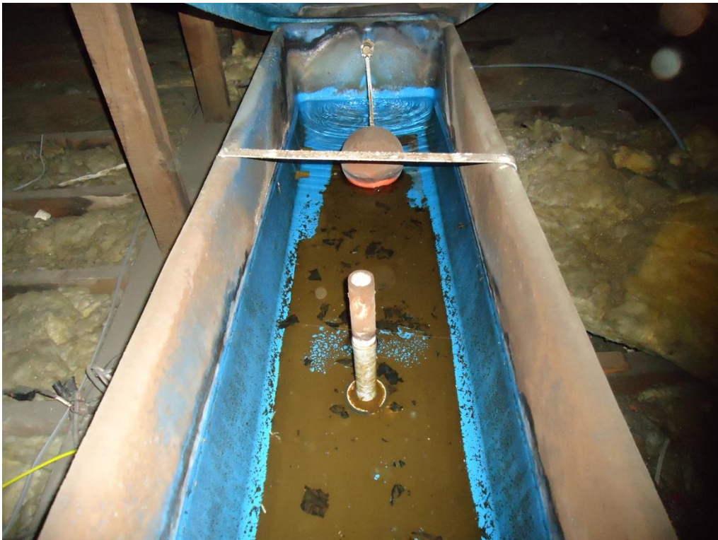
Internal condition of cold water tank
